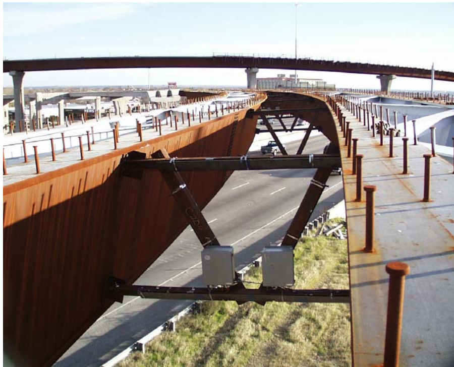
Figure 6.3 External Diaphragm #11 -- Looking South (Cheplak, 2001)
