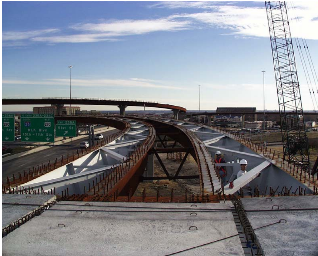
Figure 1.6 Bridge K during Construction (at 17K Looking South)
