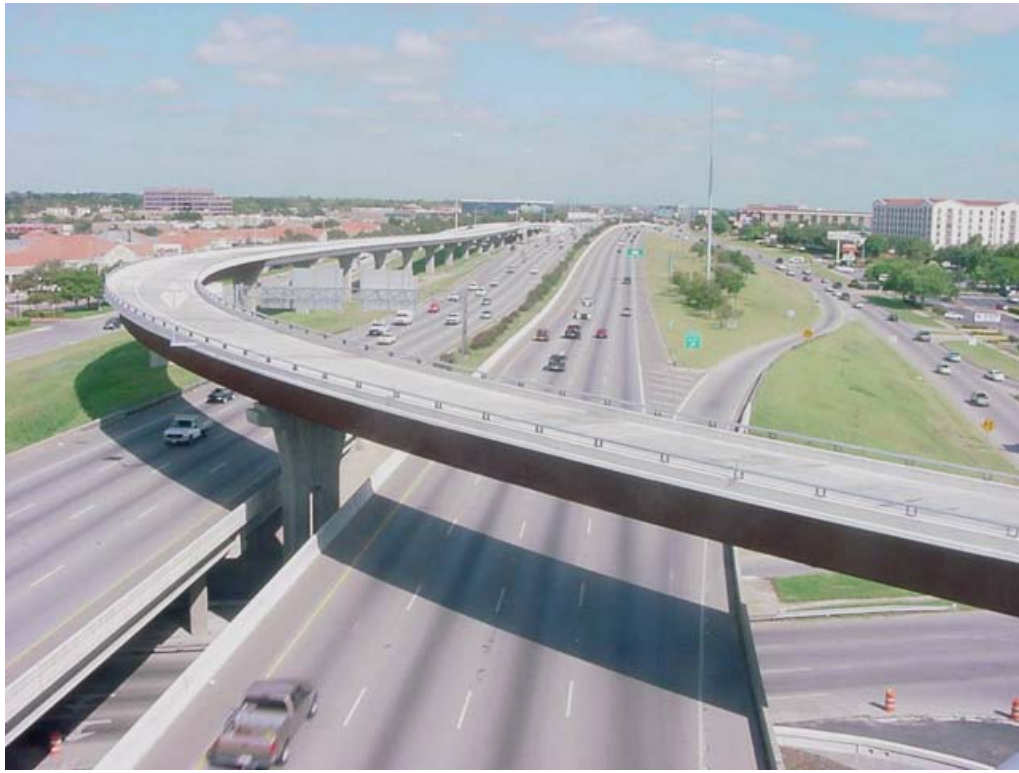
Figure 1.7 Aerial view of Completed Bridge K (Looking North)
